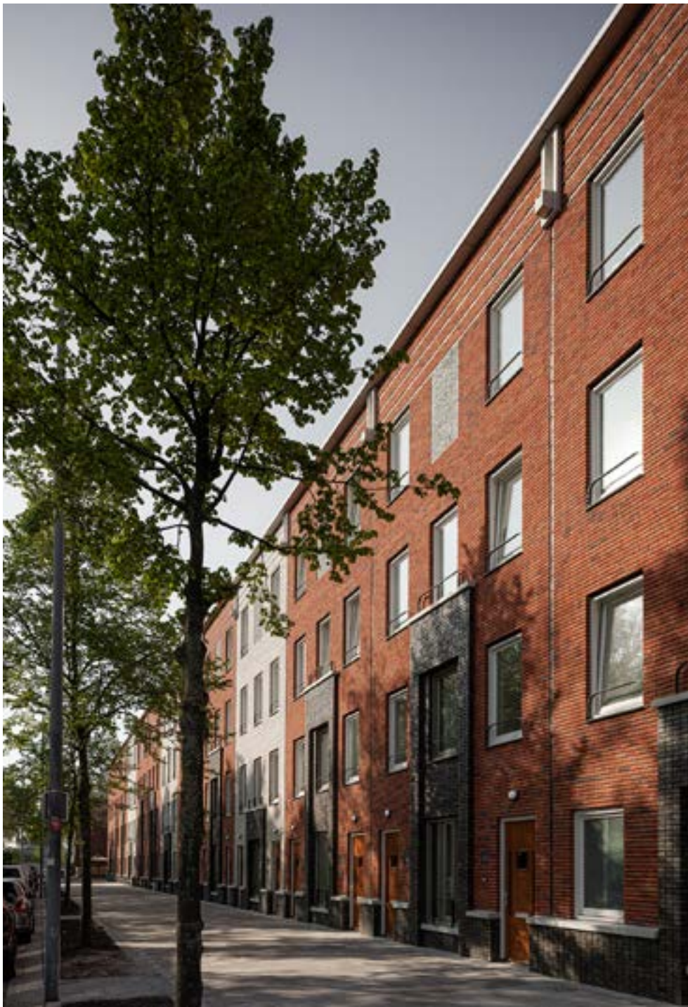
Façade along Persoonshaven (Sebastian van Damme)
