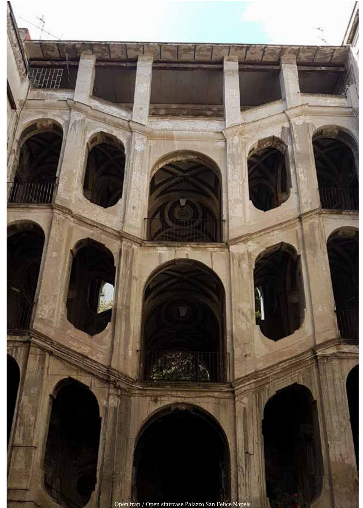
Open trap / Open staircase Palazzo San Felice Naples
