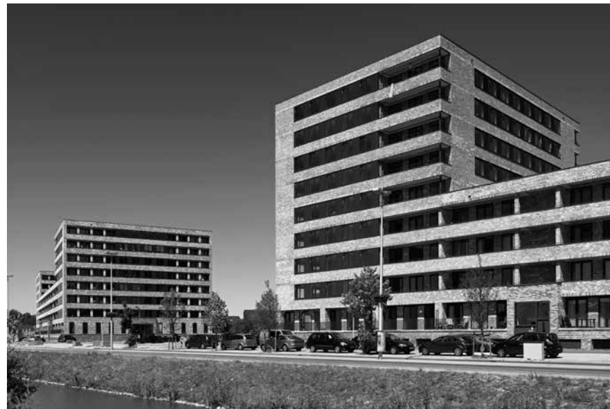
Residential buildings Langerak, Utrecht
